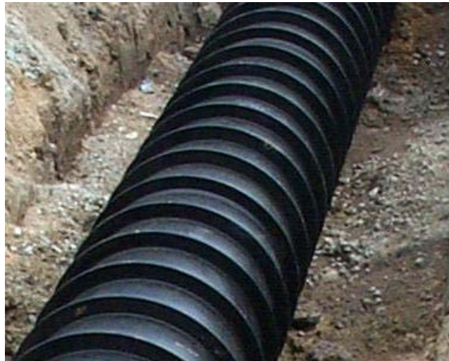
Typical RibStruct Installation
